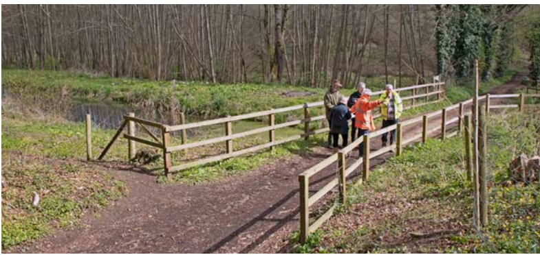
April 2022 The causeway at the site of the future Bridge 2. After a long delay thanks to Covid and planning conditions, work on site is about to start.
