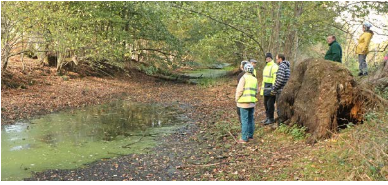
October 2018 Canal Trust volunteers and staff at the site of Bridge 1. Soon there would be a big hole in the ground here for the bridge foundations.
